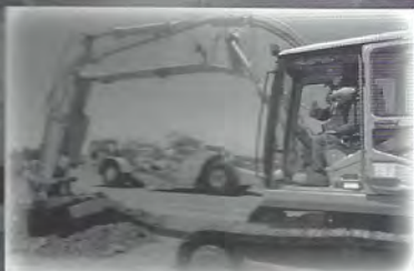
Groundbreaking for the start of construction was held May 8, 2001.
